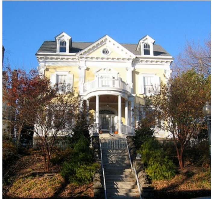
Figure 12: Recent view of Kraemer house
