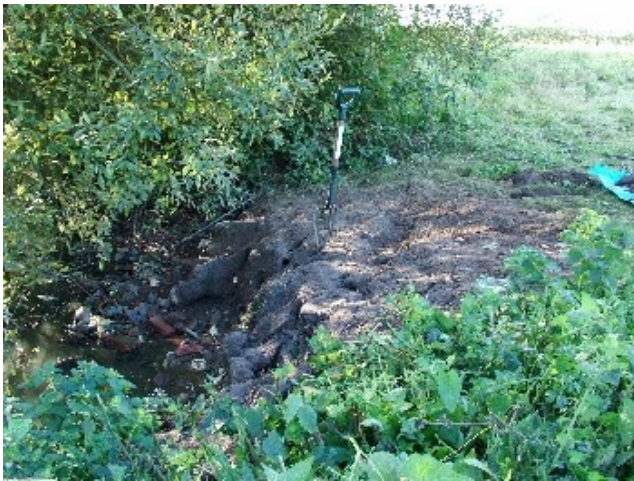
Photo 3. The Brickyard Lane tip before starting the first test trench
