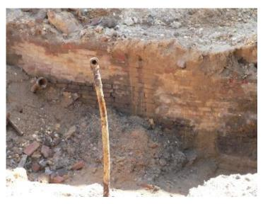
Pictures 3-4 are of construction/repairs around a pipe at Gibbon and South Royal Streets (near the Safeway, for those familiar with the area). Note that the main pipe is made of bricks.
