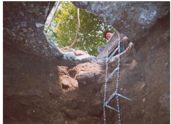
A large cavity is excavated under the concrete cap.
